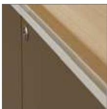
For melamine doors, recessed metal handles in matching finish to the cupboard shell
